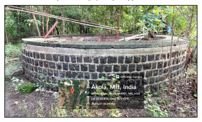
2. Bore well recharge by underground pipeline of rain water harvesting
